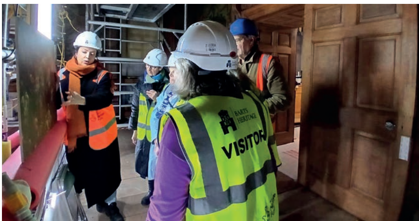
Neighbouring Histories Community Engagement group visit to the Barts Heritage restoration project
